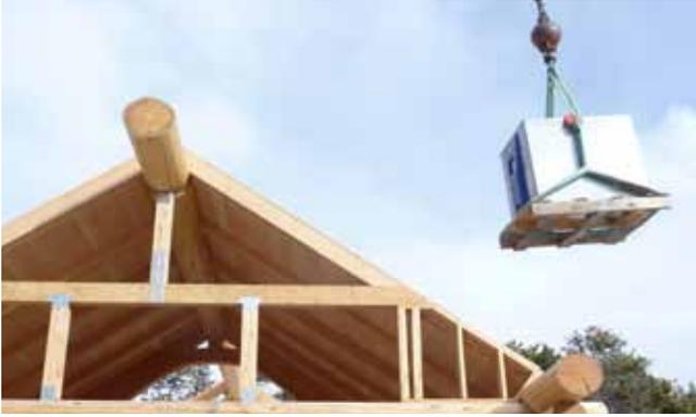
On a cabin built by Ed Shure (Timmerhus) in Nederland, Colo., the crew “flies in” the heat pump to the mechanical room.
